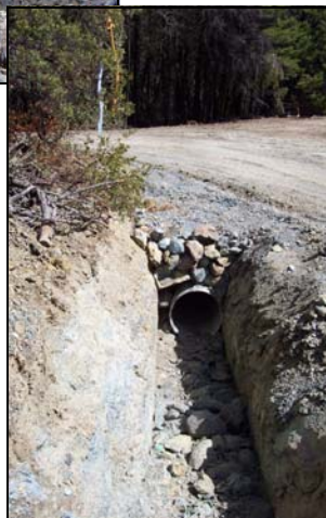
Undersized culvert was removed. The proper culvert was then installed and set at grade. The flared outlets will prevent the culvert from plugging.
